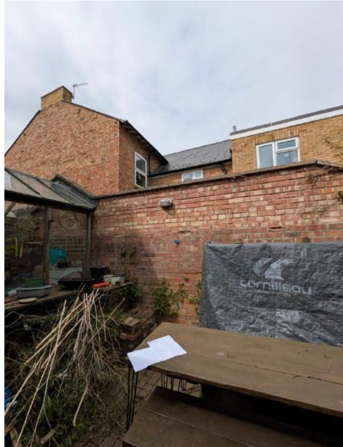
Boundary towards no.135 Hurst Street
