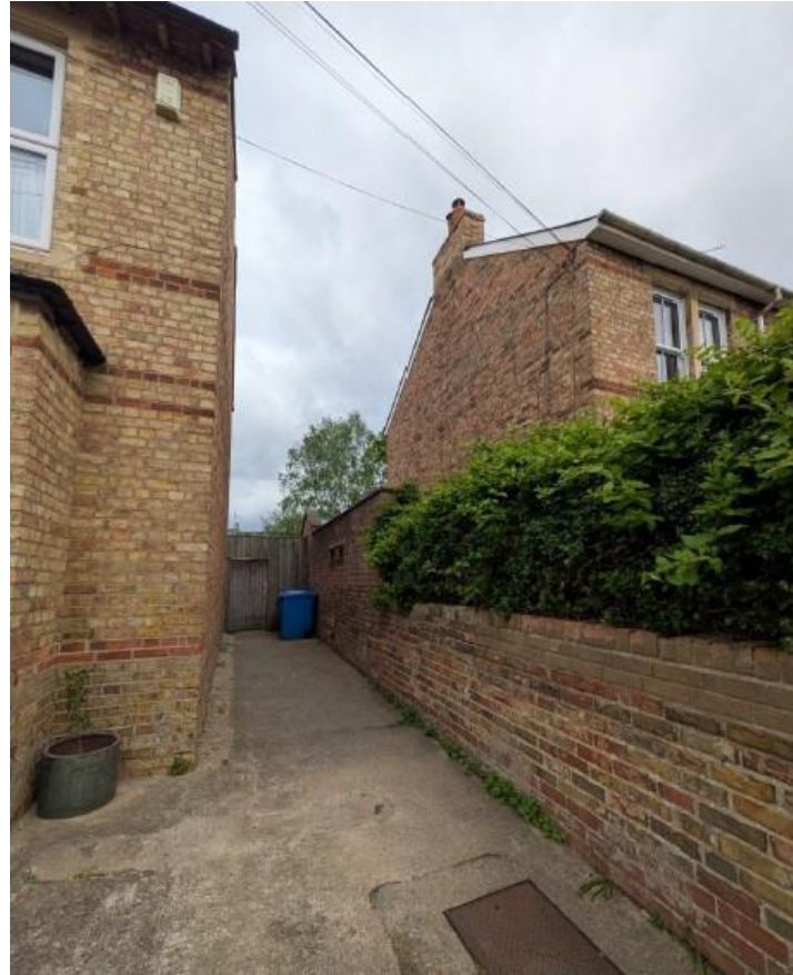
Boundary from no.135 Hurst Street (Front)
